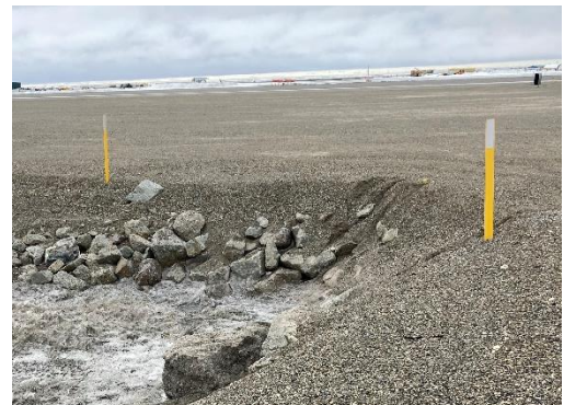
Exhibit 1 – Drainage ditch and culvert within the secured area.
